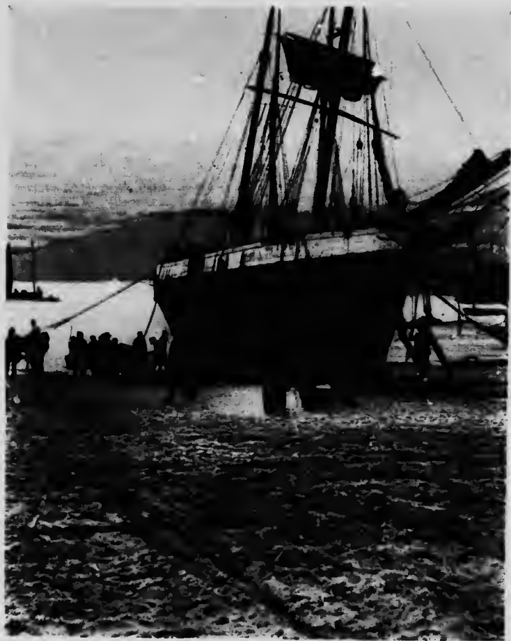
ASHORE FOR REPAIRS — ST. IVES.
